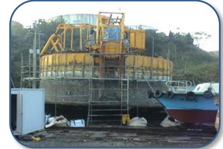
Buoy & Hose Repair
