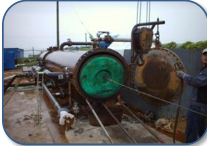
Submarine Pipe Pigging
