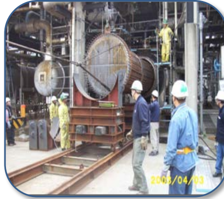
Exchanger Maintenance Work
